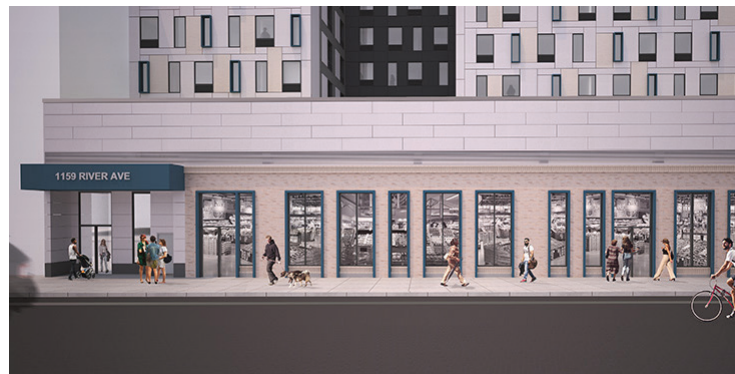
Grocery store exterior facade at the ground floor of 1159 River Avenue – Urban Quotient
